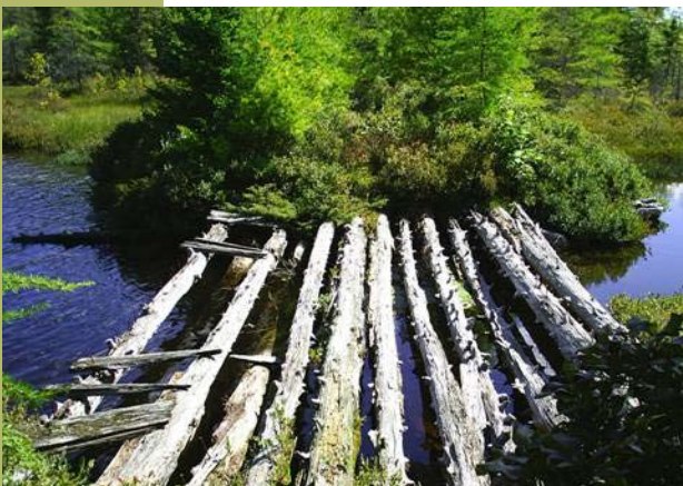
Bridges on old access roads eventually revert back to nature, like this one at Great Pine Lake (Photo by K. deGooyer)
