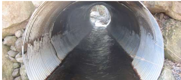
High current velocities and shallow water depths can prevent fish from moving upstream through culverts
