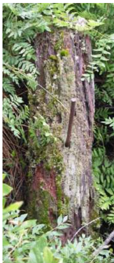
Metal spike used to secure historic timber
