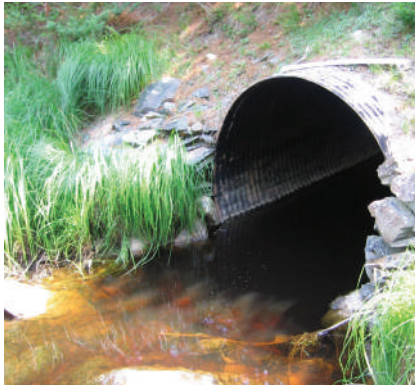
Main park road culvert at Rogers Brook, Kejimikujik
