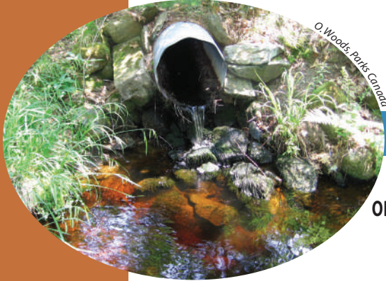
Impassable culvert for fish due to outflow drop, Canning Field Road, Kejimikujik
