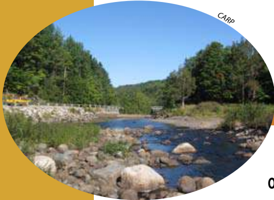
Looking downstream at the dam following the draining of the impoundment
