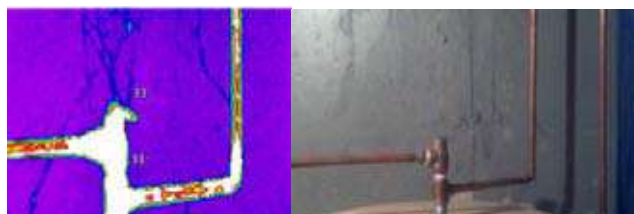
Thermal images from the top of MTRI's hot water tank show in red where heat is escaping and insulation could save energy
