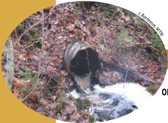
Rogers Brook culvert, which is impassable to fish due to outflow drop
