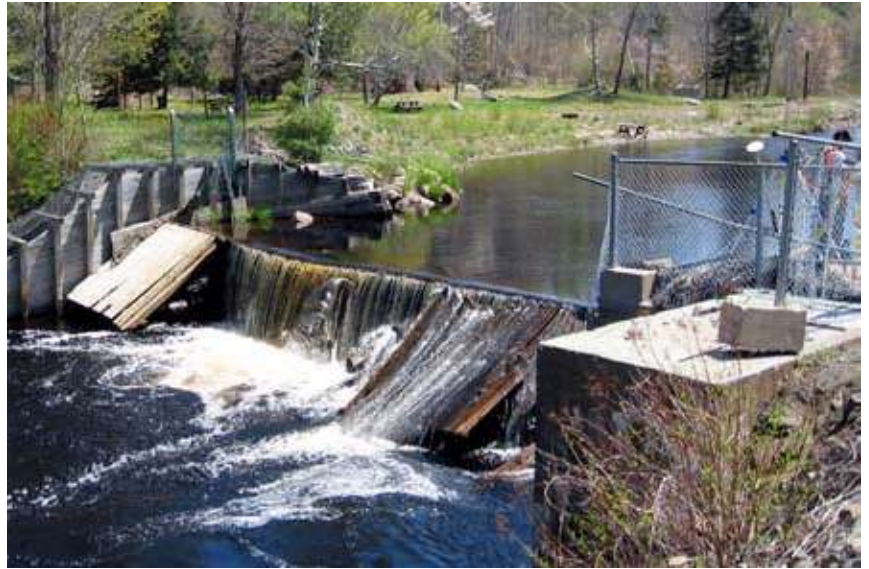
Note the deterioration of the spillway when looking upstream at the Clementsport dam in May 2009
