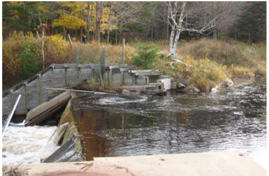
Clementsport dam, October 2009, with whirlpool above hole in toe of dam
