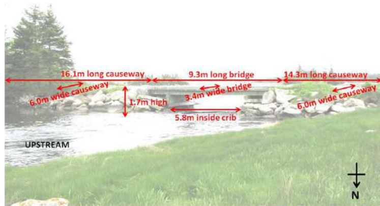
New bridge dimensions showing the restricted flow through the narrowed channel
