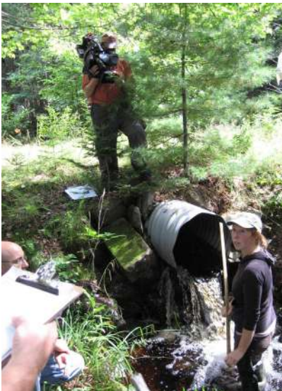
Perched culvert on the Canning Field Road
