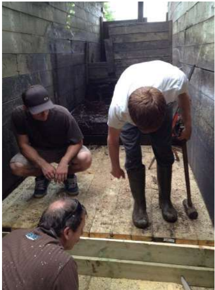
Students working on the floor of the fish ladder
