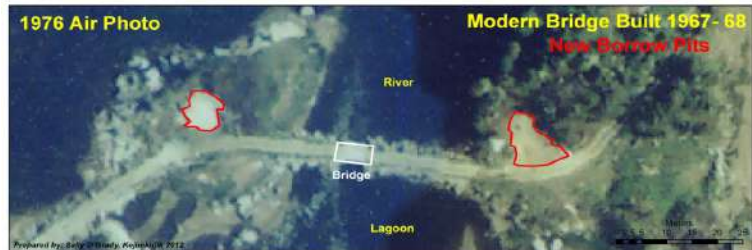
Aerial photos from 1965 and 1976 showing older bridge span with posts and new shorter bridge with earthen approaches completed in 1968
