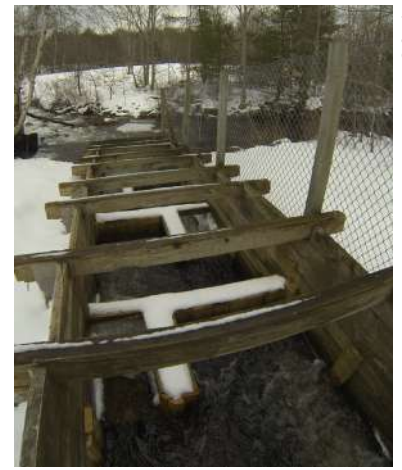
Harmony fish ladder functioning in the late winter
