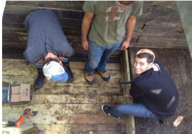
Continuing construction of the fish ladder
