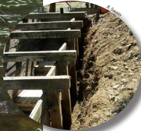
Harmony fish ladder's outer wall completely excavated
