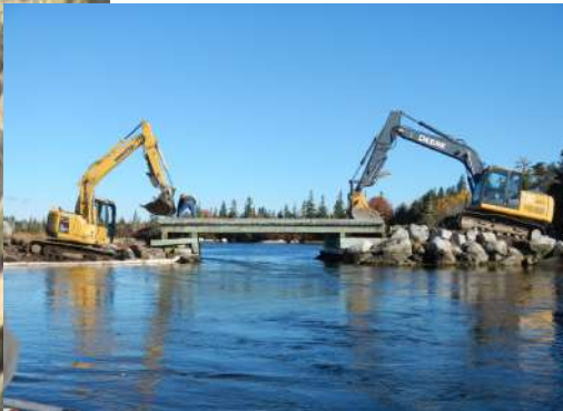
Excavators moving the bridge
