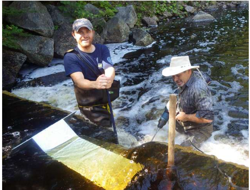
CARP and NSLC Adopt A Stream staff installing a fish chute at the outflow of a barrier culvert
