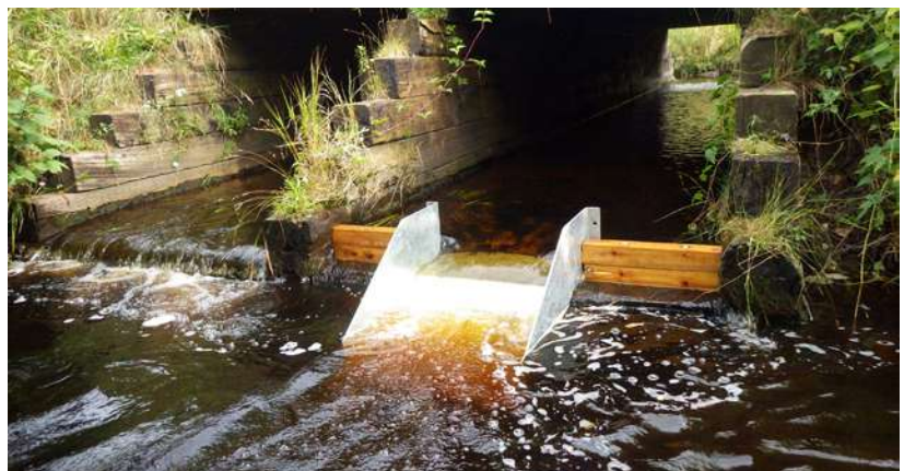
A fish chute, installed as part of restoration initiatives to restore fish passage
